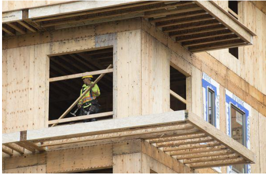
Housing construction in Vancouver. JONATHAN HAYWARD/THE CANADIAN PRESS
