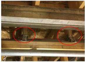
Crushing and twisting of truss bottoms were noted by inspectors who were tasked with investigating the damage caused by a fire on the property. (Read Jones Christoffersen Ltd.) Rose Ferris, who has owned a unit in the building for 23 years and sits on the condo board, was packing up boxes on Tuesday.
