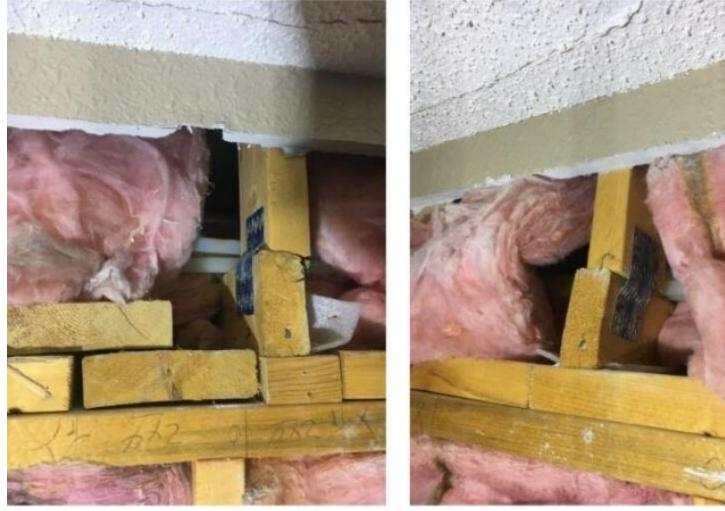
Images gathered by engineers demonstrate some of the framing issues uncovered during various inspections of the building. (Read Jones Christoffersen Ltd.) Thurber said the city will be monitoring the situation, and if the appropriate action isn't taken, it has authority under the Safety Codes Act to take enforcement action against the building owners.
